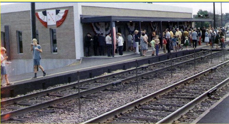
Looking to the east – April 1971
