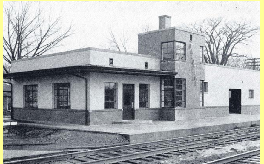
This structure, opened in February 1949, was replaced in April 1971.
