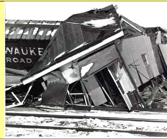
This is the tower at about 12:00 noon on 02/05/1978
