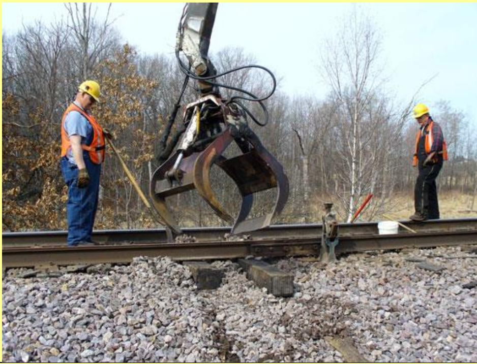
Foreman Leroy Sprinkle and Layton Wahlberg , replacing some ties just east of Fairchild, WI in April 2007. Photo by Louis Wilson .
