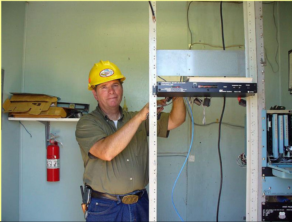
Radio Technician Jeff Phillips installing a new radio at the Humbird, WI hot box detector on 07/27/07. Jeff works out of Butler and has 31 years of C&NW & UP service. Photo by Louis Wilson .
