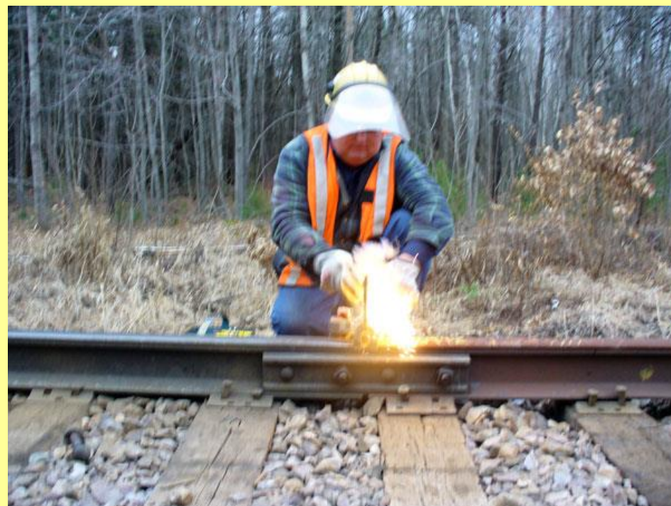
Signal Maintainer B.J. Bruhling flashing on a bond wire between Altoona and Fall Creek. BJ works out of Altoona and has over 30 years of C&NW and UP service. Photo by Louis Wilson .
