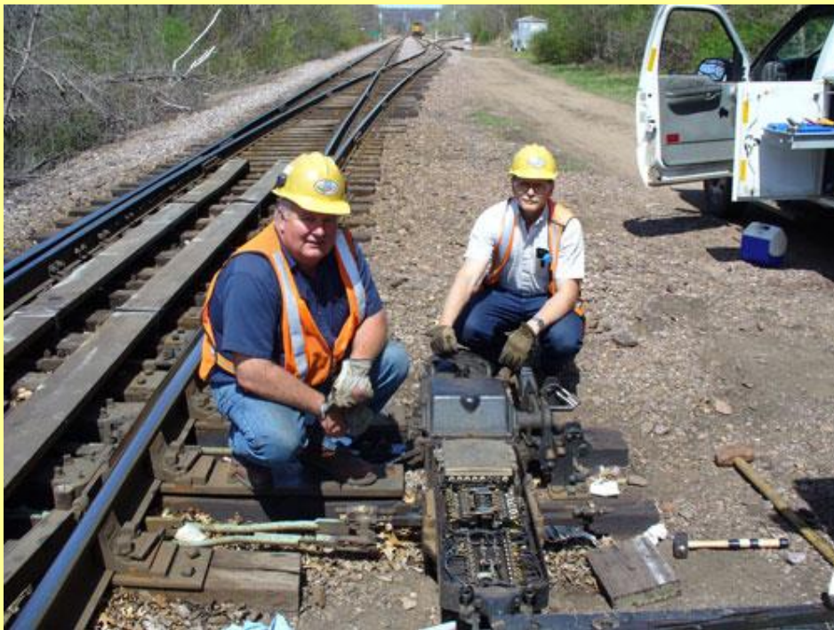
Benny Bruhling and Jim Lapcinski adjusting a power switch machine at Yukon Jct., Eau Claire, WI during April 2007. Both started with the C&NW and have over 30 years of service. Photo by Louis Wilson .
